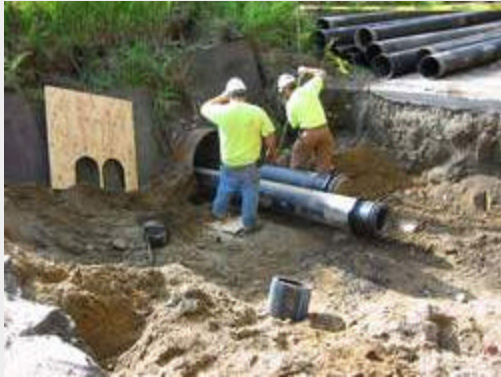
Correspondent photo by Jessie Salisbury Workmen insert the second water pipe.
